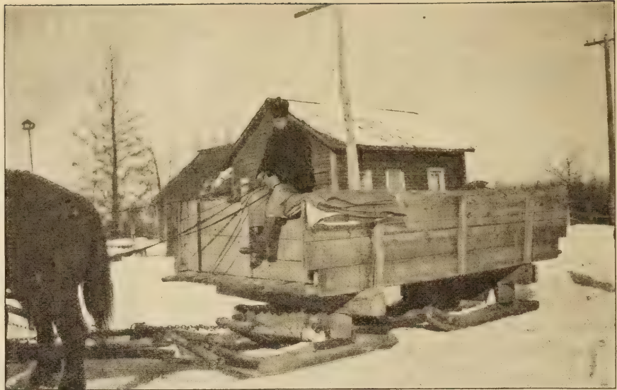
HAULING GRAVEL IN WINTER FOR ROAD WORK. LOAD OF SIX CUBIC YARDS HAULED BY TWO TEAMS 7\frac{1}{2} MILES, OVER GRADES UP TO 6 PER CENT.
